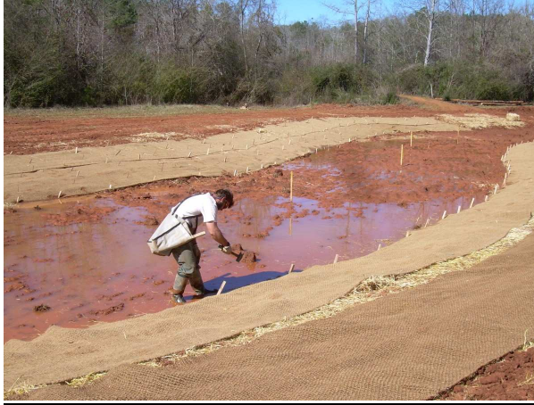
Fig.1-Two types of coir blankets stabilize banks of stream in Georgia
