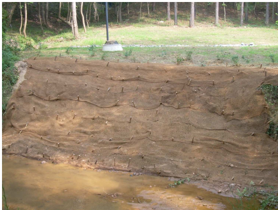
Fig.2-Coir blankets protect South Carolina streambanks
