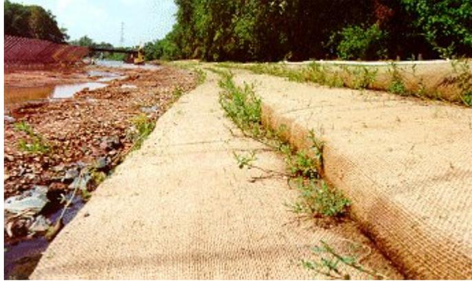
**Figure 1: Bioengineered river bank stabilization, an innovative fabric-encapsulated technique.**
